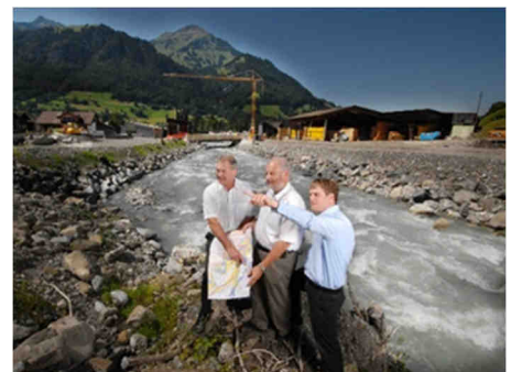
Flood protection measures in the Reichenbach, one of many prevention projects.
